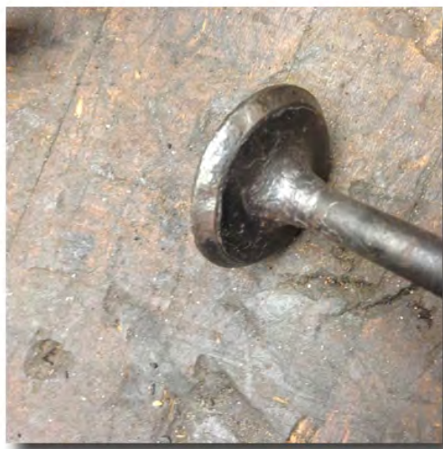
This valve is burnt and leaking
